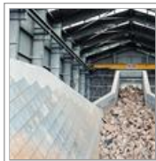
Crushing circuit benefits from early contractor involvement
